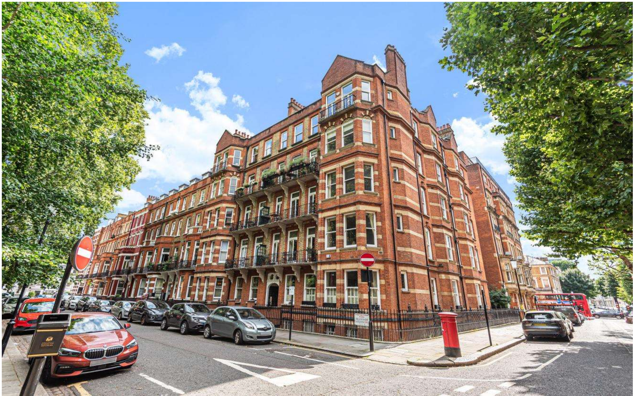
Bramham Gardens, Earls Court, SW5
