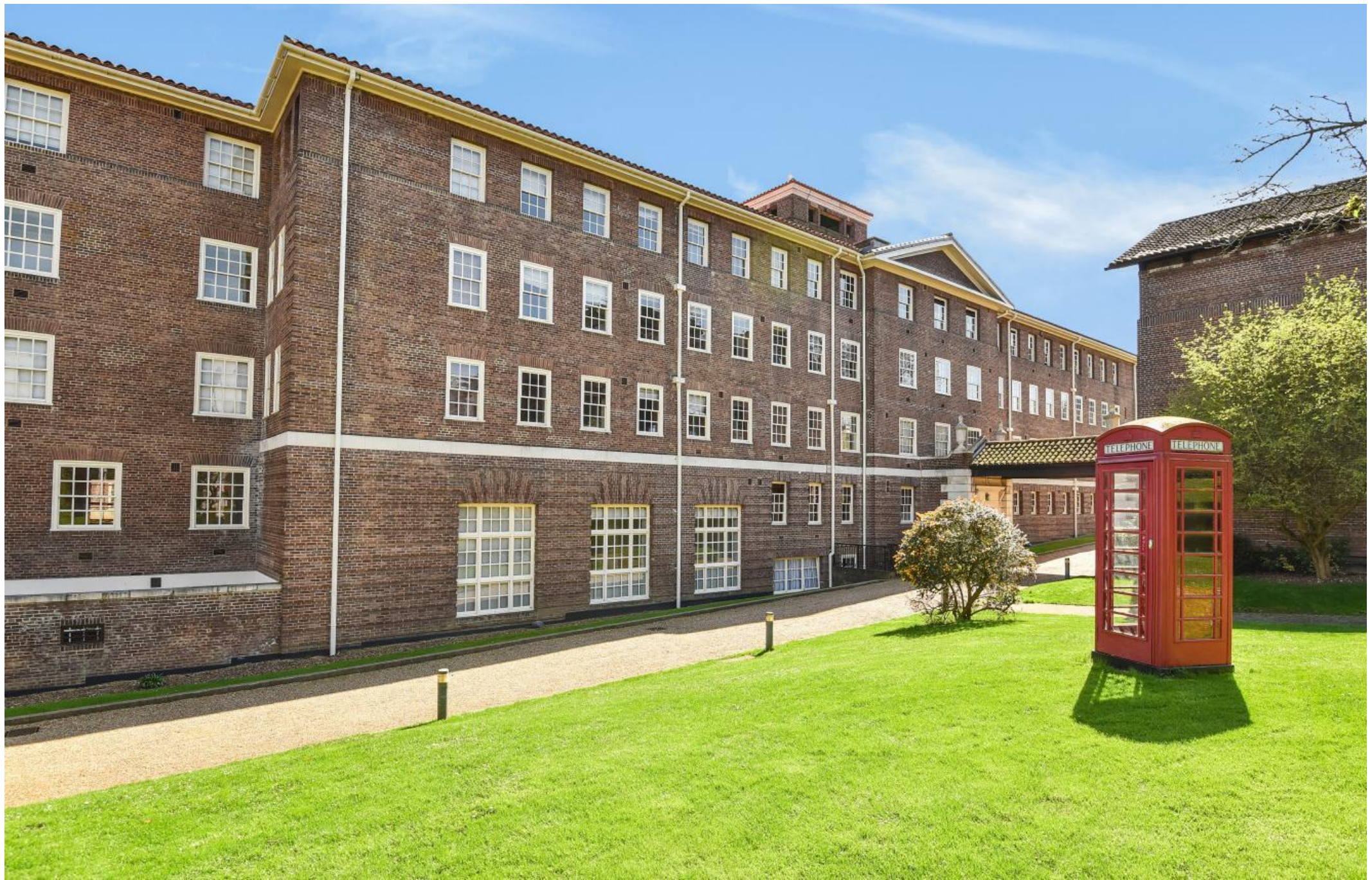
Scott Avenue, Putney, SW15
